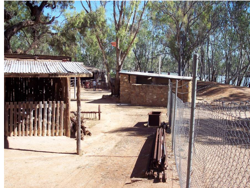
Fences visible from the Riverfront Focal Point are to be replaced.
