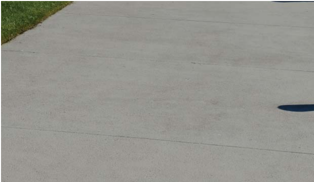
Washed Aggregate Paving Footpaths
